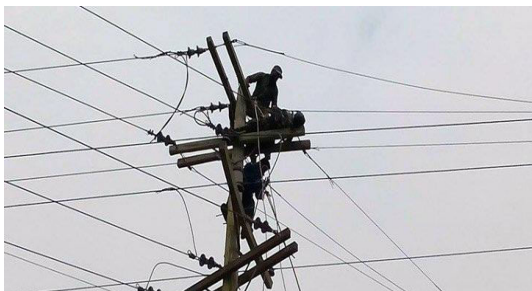
Fig.1.1 : Electrician at Work
