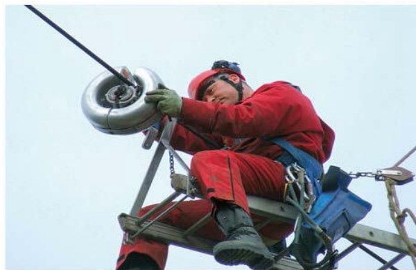
Fig 2.installation of power donuts
