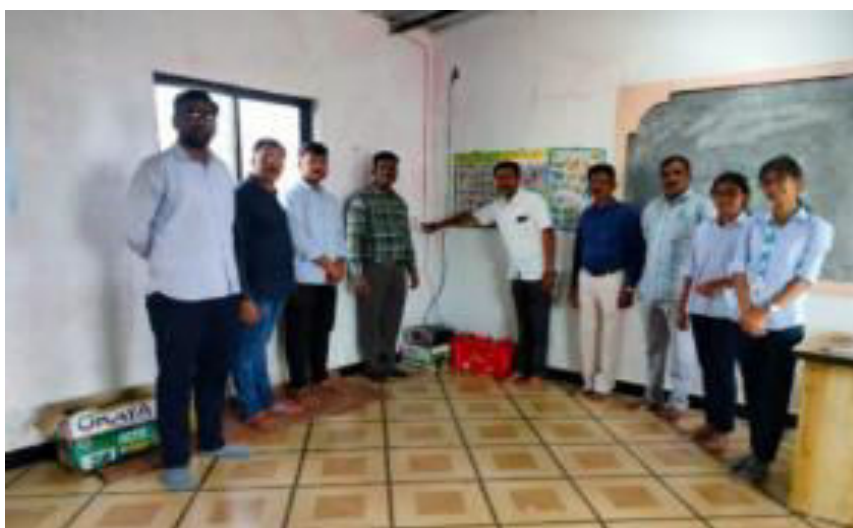
Fig.6 .Successfully installation of PV panel system in rural Elementary School Bamberwadi
