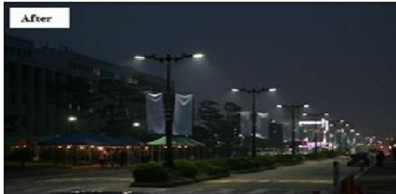
Figure.8 Realization of Smart LED lighting system.
