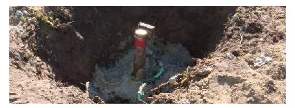
Fig 3.Bentonite Earthing
