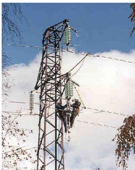
Figure 7 Photograph installing line surge arresters
