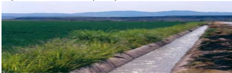
Concrete Lined Canal
