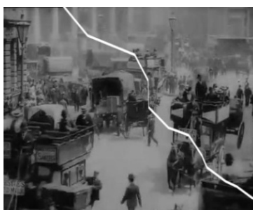
Fig. 1Example of a Frame Damaged by Tear
