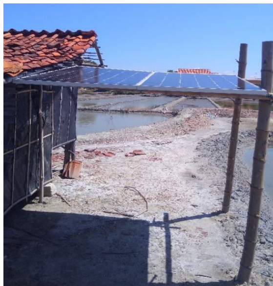
Fig 3. Solar Panel Contruction
