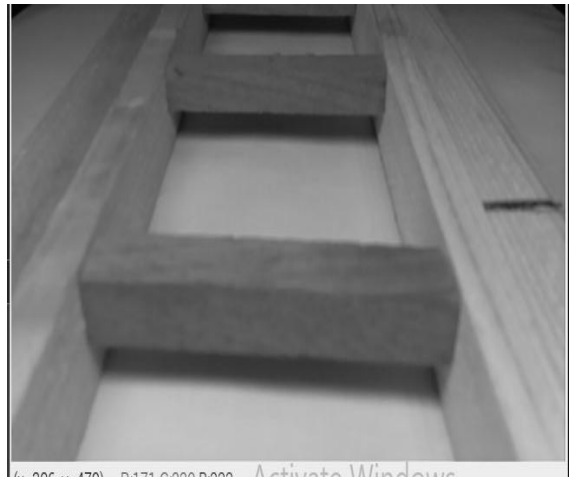
Fig 5: Gray Image of track with crack
