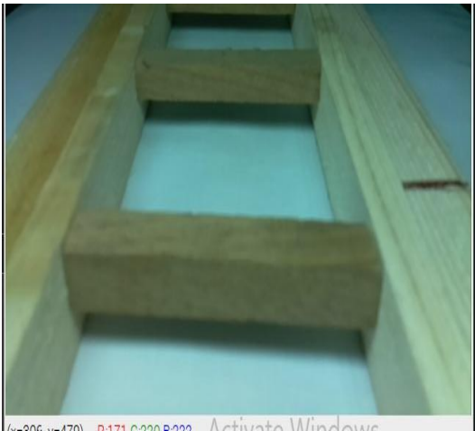
Fig 4: Original Image of track with crack
